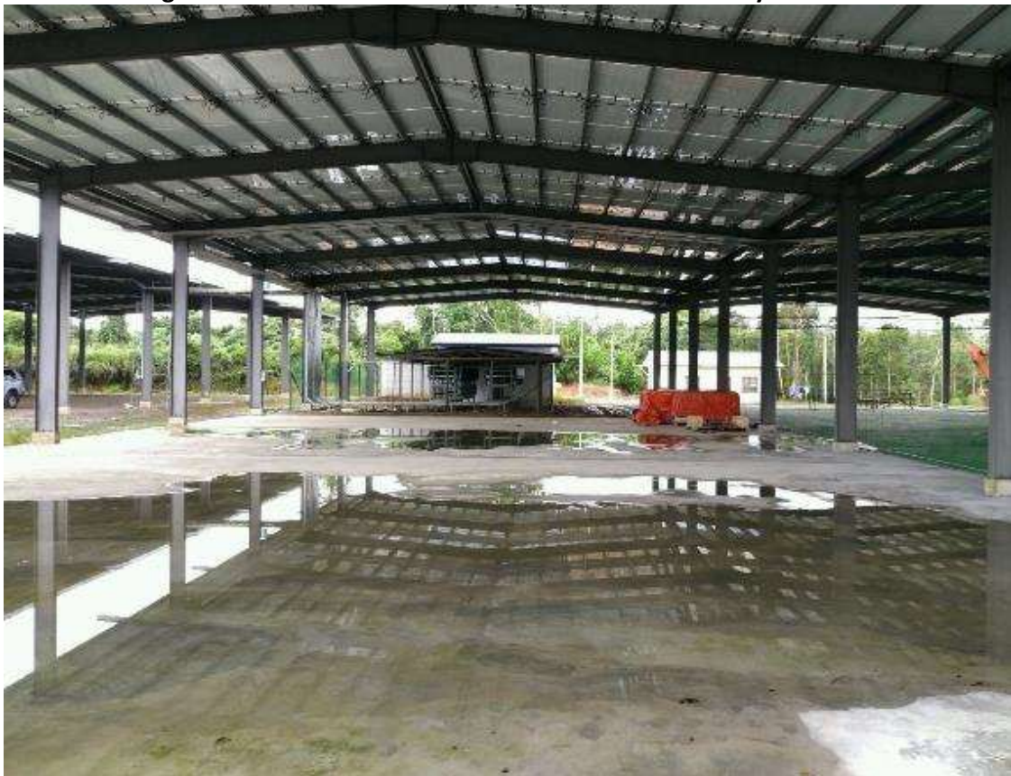
Figure 33 - The Ground Below The Structure Is Not Fully Utilized (And Concrete Floor Is Wet Maybe Due To Roof Leaking)
