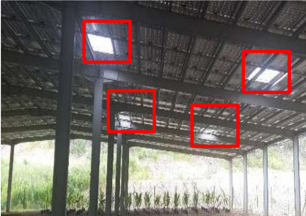
Figure 15 - All PV Arrays MUST BE COVERED. Sunroofs Can Be Installed To Allow Penetration Of Sun.
