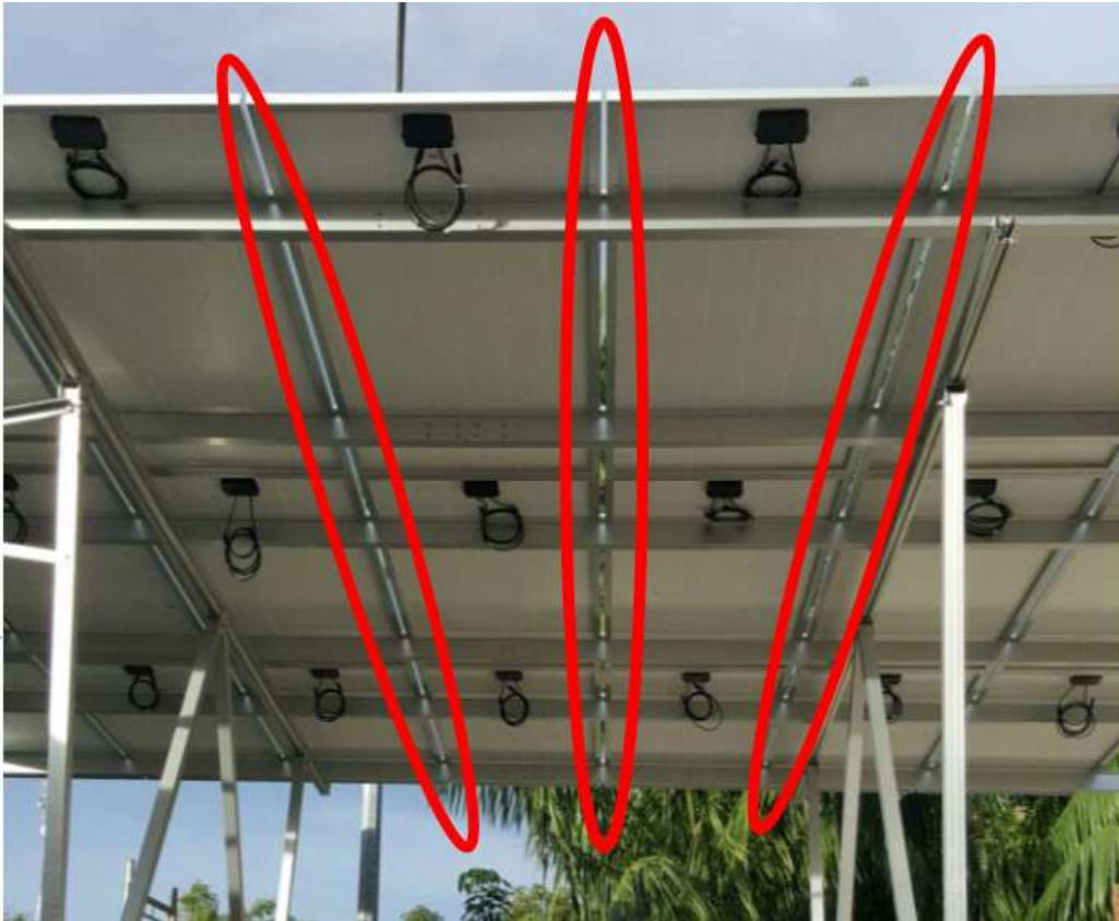
Figure 13 - Gaps Between PV Modules Are NOT Allowed
