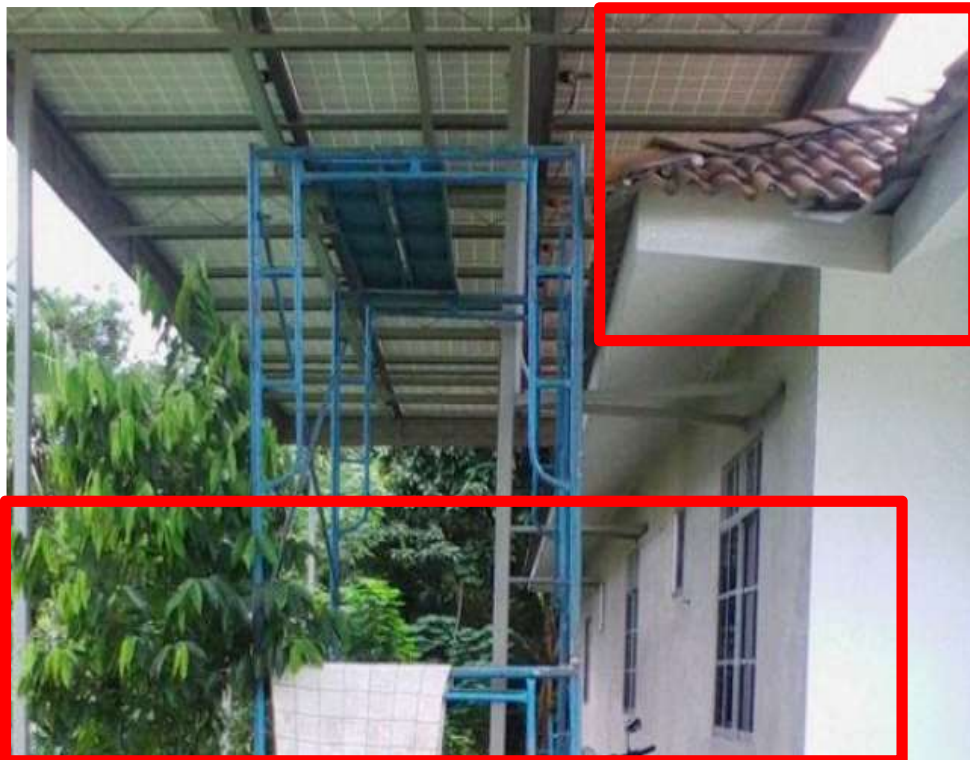
Figure 11 - Overlapping Of Modules On Top Of Existing Roof & Using Inappropriate Construction Materials
