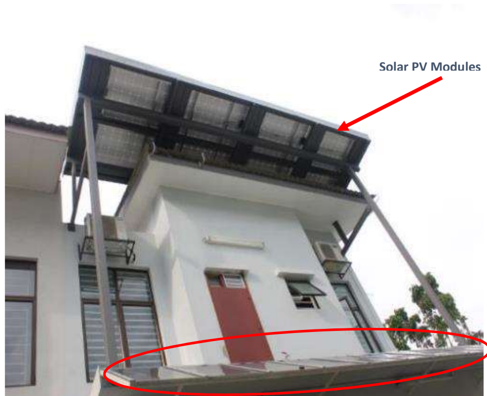
Figure 4 - A Secondary Roof Beneath The Modules Serving The Same Function
