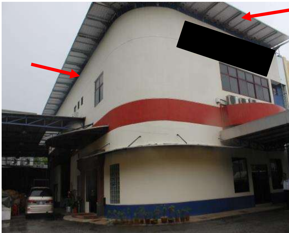
Figure 16 - Installation serves no function or purpose (PV Module Too High to Serve as Roof)
