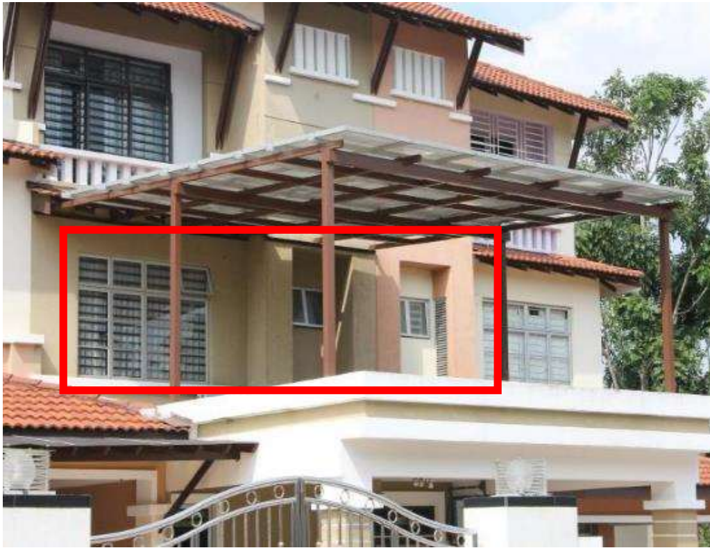
Figure 8 - No Access Door As To Serve The Function Of Installation As A Balcony
