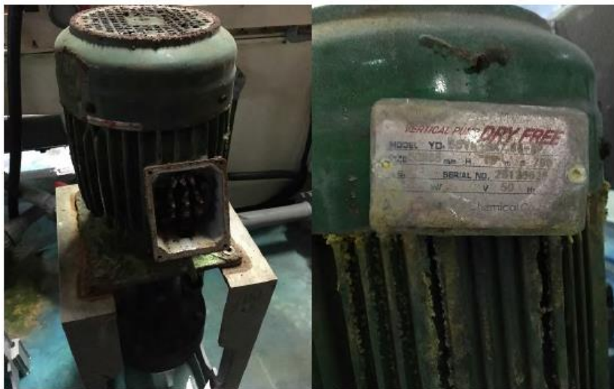
Figure 4-23 Corroded Motor at Etching Line
