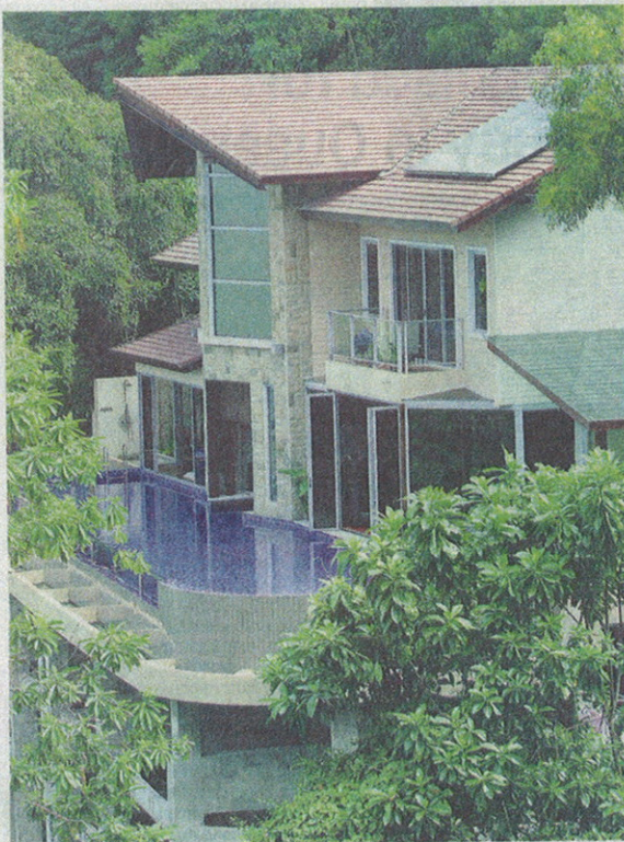
Generating income: The solar photovoltaic panel atop the roof of Tan's bungalow.
