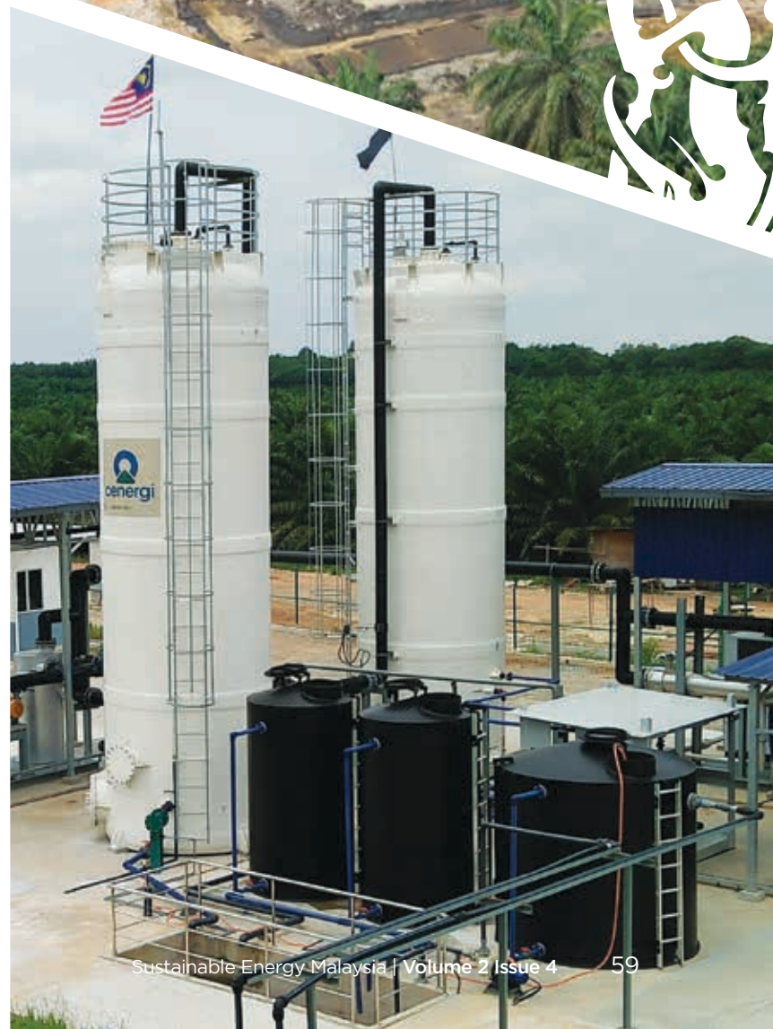
Sri Jelutong's Biogas Power Plant utilises two scrubbers; one for main operations and the other serves as backup.
