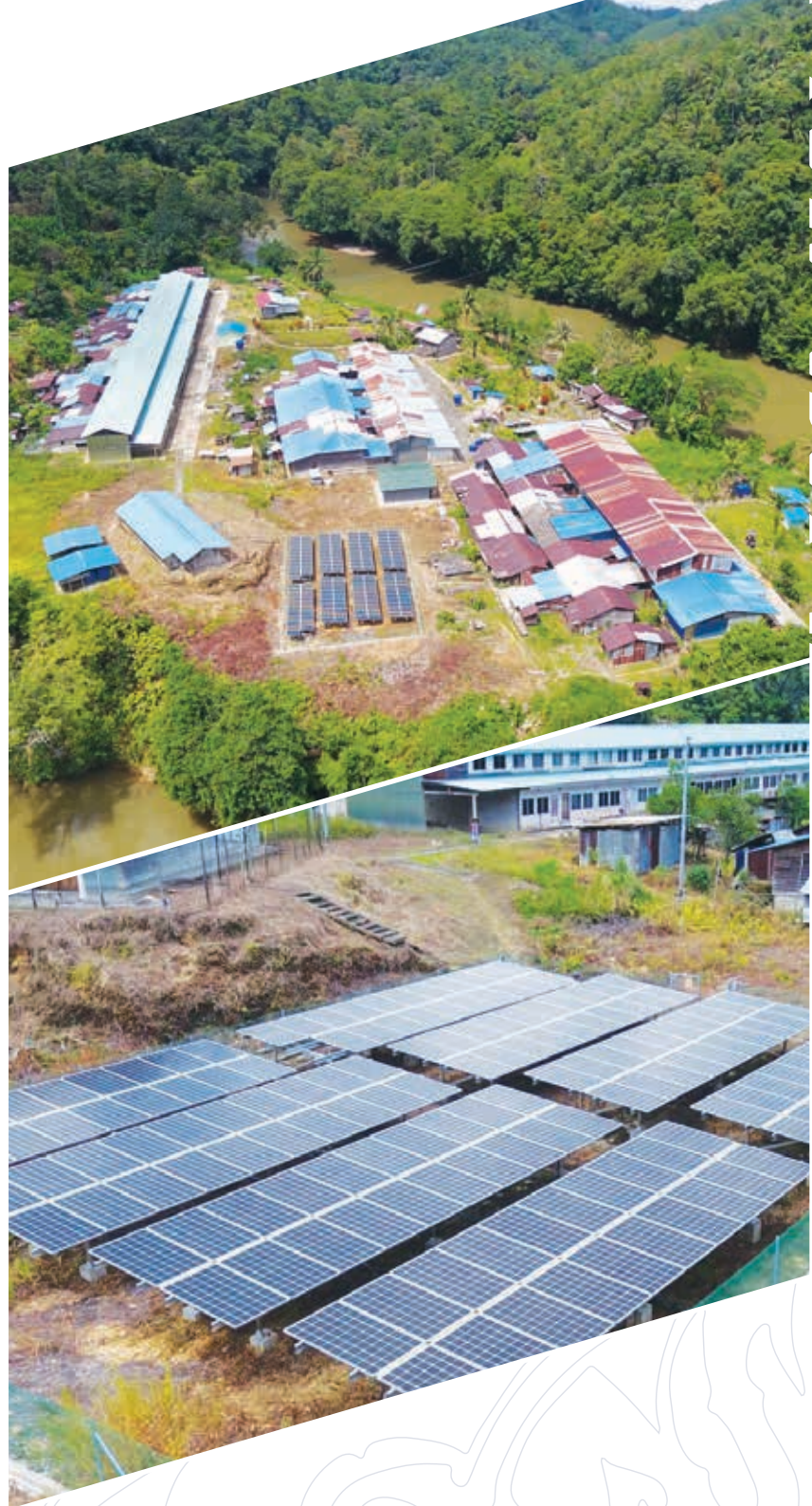
↑ A standard Centralised Solar System under SARES.
