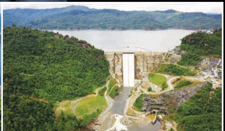
⬆ The 944-MW Murum Hydroelectric Power Plant.
